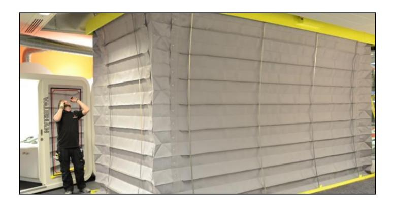
Fire Curtains are installed to enhance the fire protection abilities at Coda. The locations of the fire curtains are on the 10<sup>th</sup> and 11<sup>th</sup> floor atrium in the East Tower as well as the 9<sup>th</sup> through the 13<sup>th</sup> floor interior stairwells in the South Tower.
