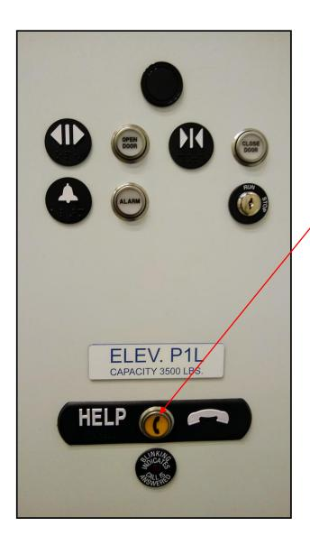
Each elevator is equipped with a Help Button should you experience a problem with the elevator. The Help button is monitored 24/7 by a Thyssenkrupp (TKE) Elevator offsite monitoring facility.
