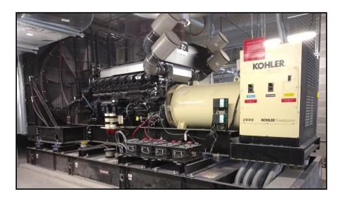
The emergency generator can provide 11 hours of emergency power at 75 percent load.
